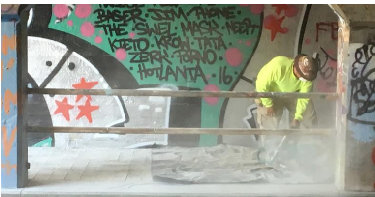
Paver installation in Krog Tunnel
