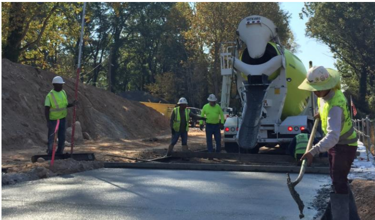
Concrete paving on the northern end of the Westside
